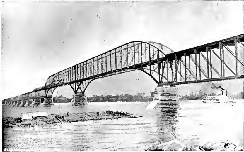
ST. LAWRENCE BRIDGE. C. P. R. LACHINE.
